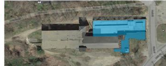
Aerial Highlighting Subtracted Structures
